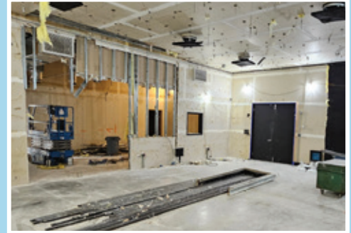
Mid-construction with mechanical, electrical, and plumbing being removed.
