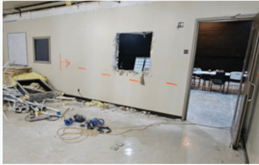
Demolition of the control room, looking into the studio.
