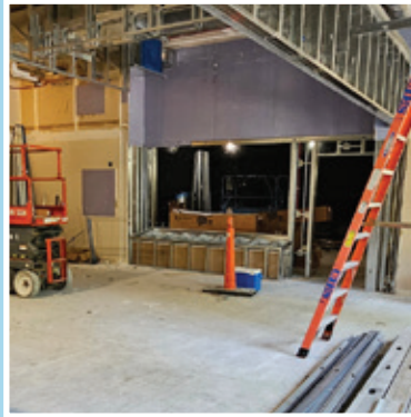
New walls being built and mechanical, electrical, and plumbing reconfigured for higher ceilings. View toward newsroom (left) and toward studio (right).
