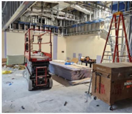
New walls being built and mechanical, electrical, and plumbing reconfigured for higher ceilings. View toward newsroom (left) and toward studio (right).
